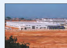
Hunter Douglas Construction Elements, Xiamen, China
