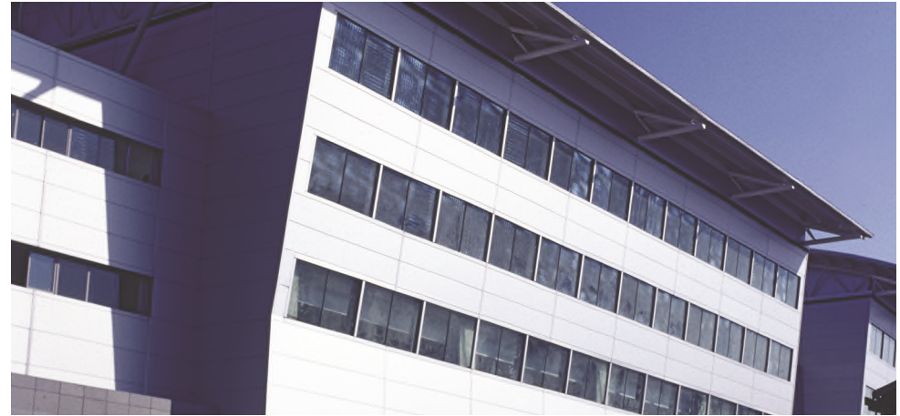
Changchun Railway station, China
