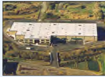
Hunter Douglas Fabrication, Renton (WA), U.S.A.
